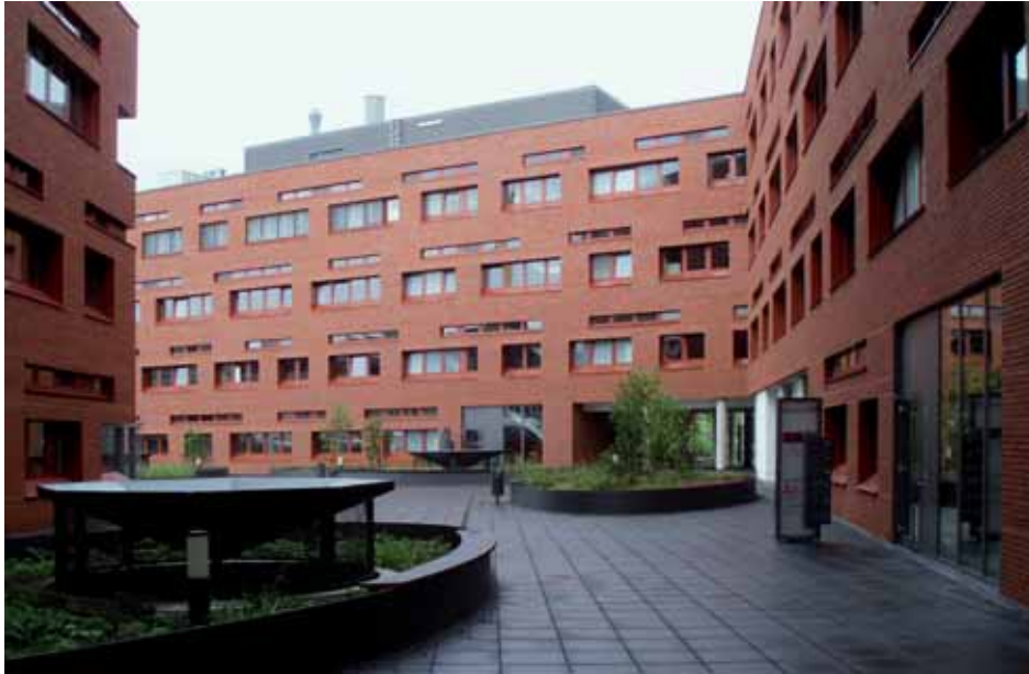
Inner courtyard of the BIO CITY.
