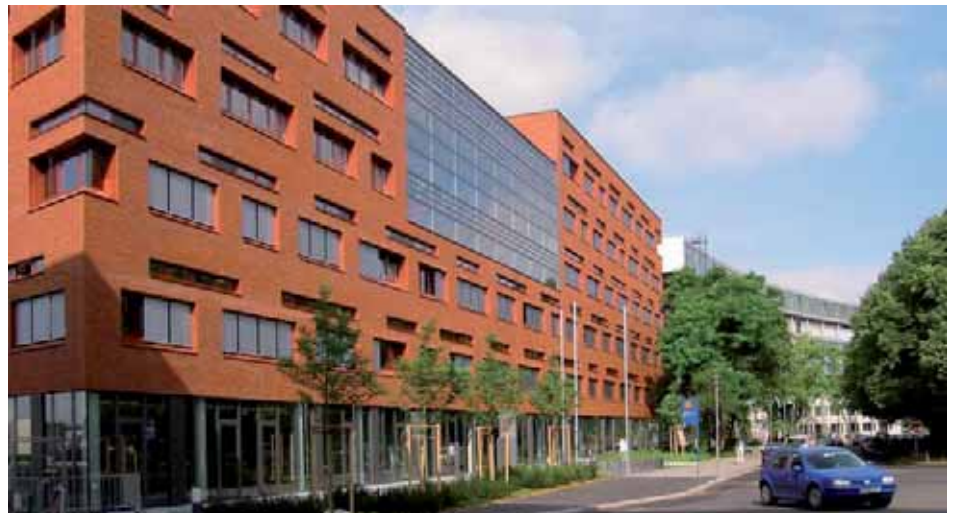
The new building of the institute during construction in April 2007 (above) and the BIO CITY (below).
