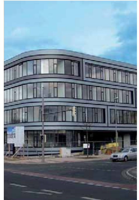
View on the new building, status april 2007.
